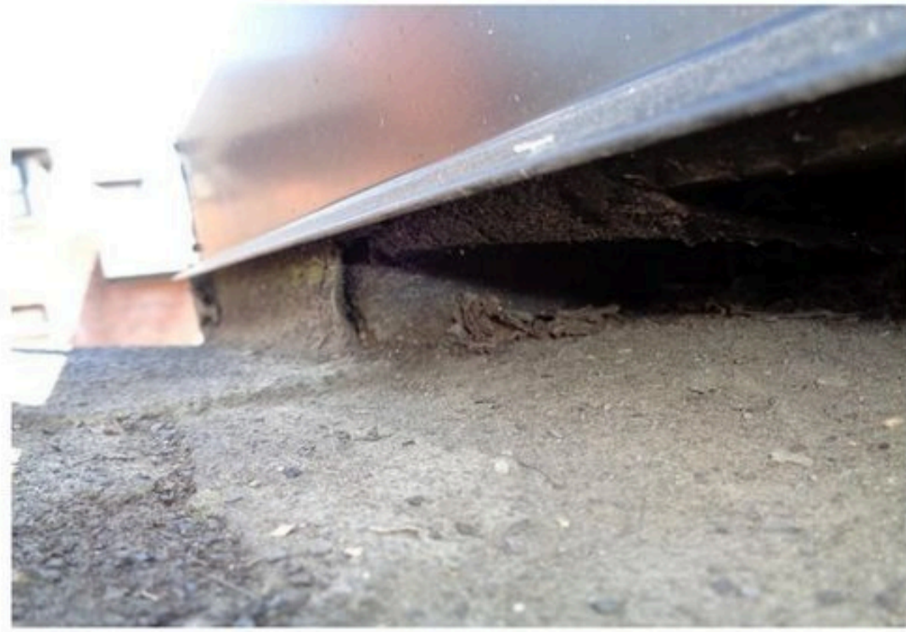
Image 007 and 008. Shingle to membrane tie-in. Membrane not adhered to the drip edge.
