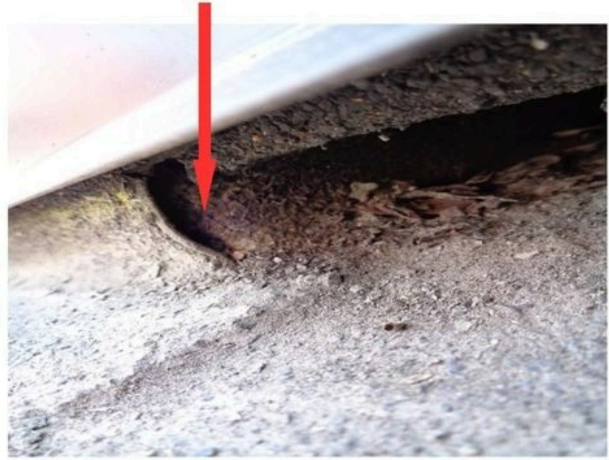
Image 007 and 008. Shingle to membrane tie-in. Membrane not adhered to the drip edge.
