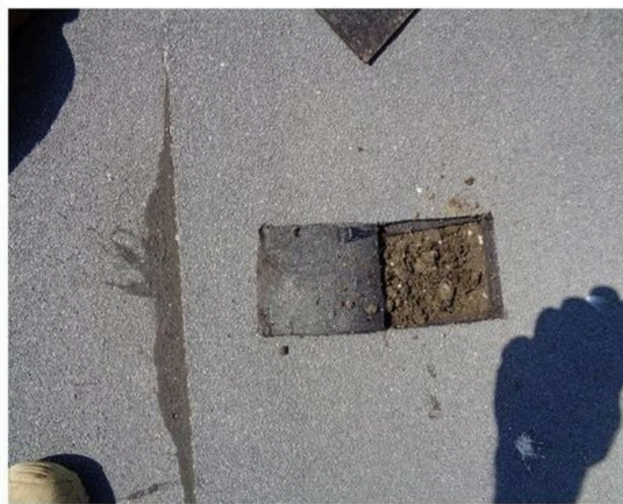
Images 001 and 002. No new insulation. Wet 4-ply ply felt membrane (tar and gravel) still in place.
